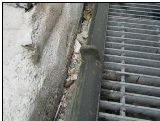
Photos showing the gap between concrete kerb on the track littered with debris and litters
