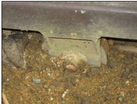
Photo showing one the wheels of the incident stuck in soft ground
