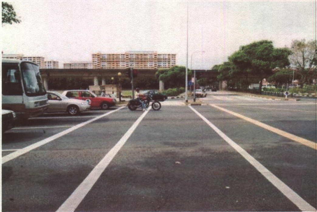
Figure 1: Existing pedestrian crossing lines
