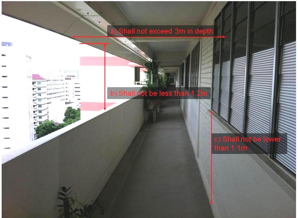
**Pre-1990 HDB layout where relocation of gas meter is permitted/not permitted**
