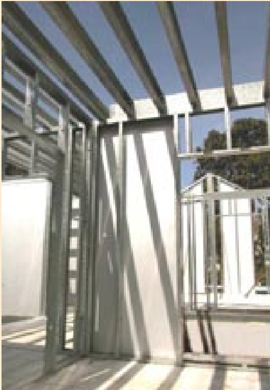
Close-up of the second storey prefabricated structure.
