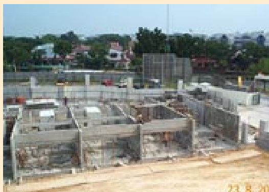
Precast works at Goldenhill Villas.
