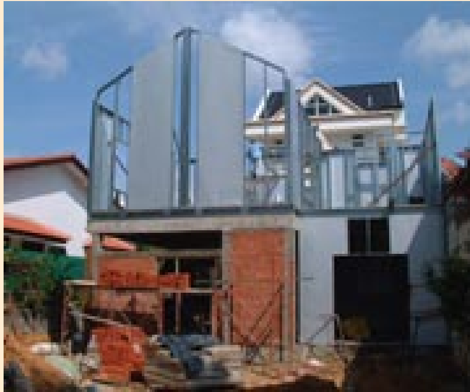
The lightweight steel panels were prefabricated in the factory.
