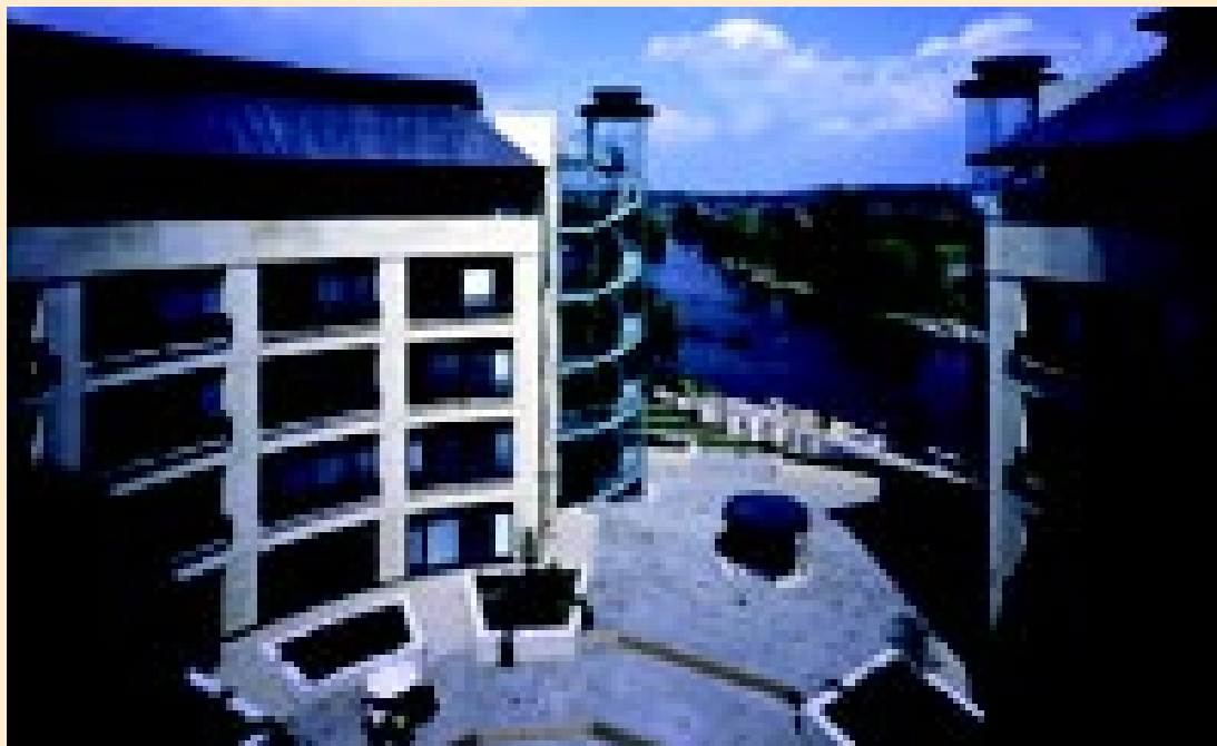
The benefits of both in-situ and precast concrete were fully exploited at Thames Water's new HQ in Reading.
