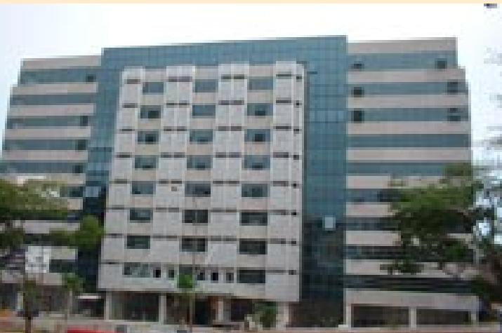
Polished reconstructed stone façade at the E-Centre.
