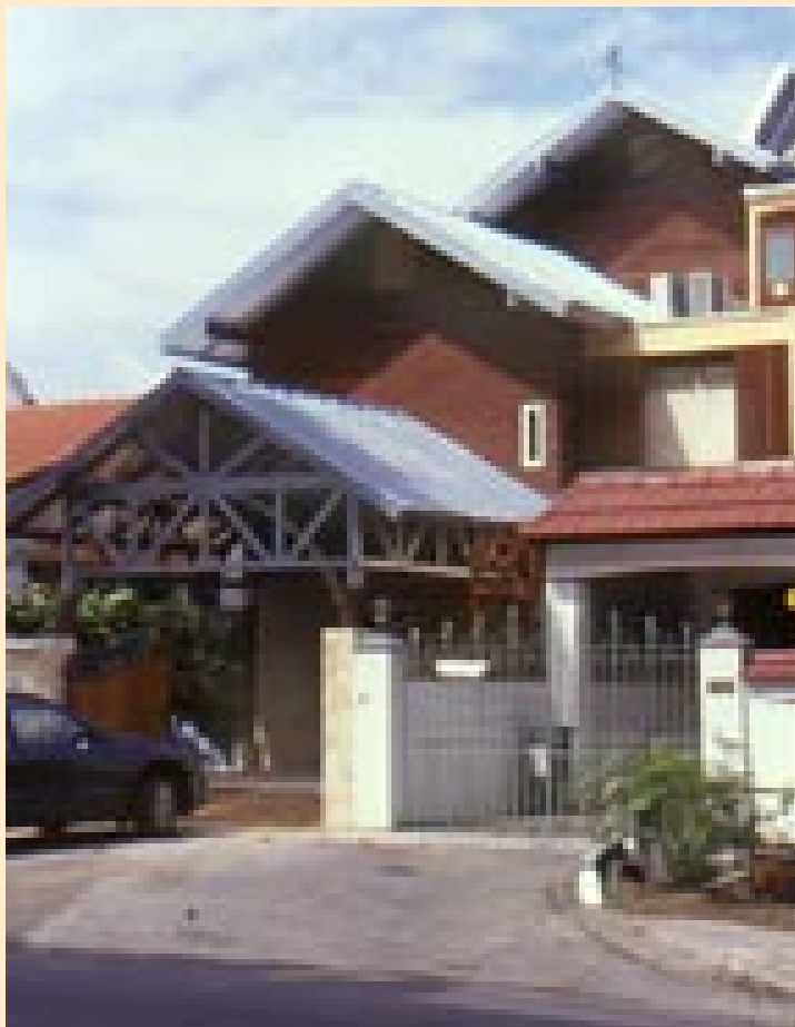
The completed house.
