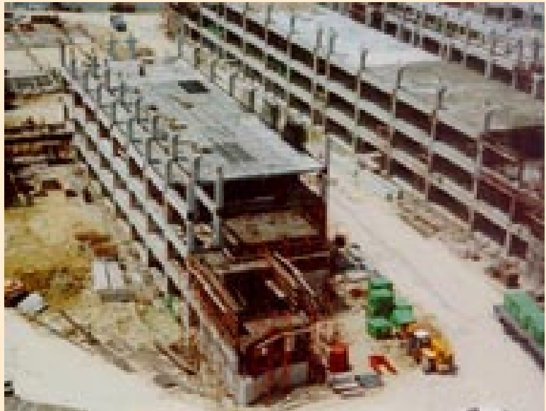
Precast elements installation at Bedok Green Secondary School.
