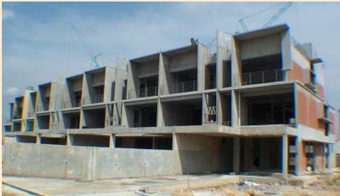
Goldenhill Villas- construction using precast technology.
