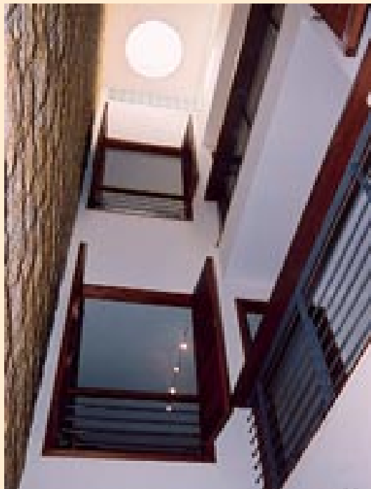
Interior air-well looking up towards skylight and turbine ventilator.
