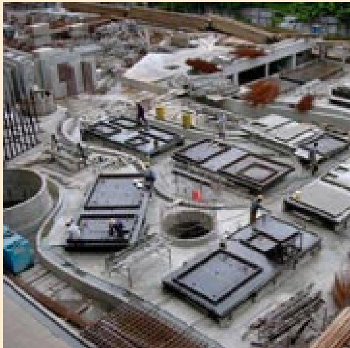
Precast façade panel casting operation.
