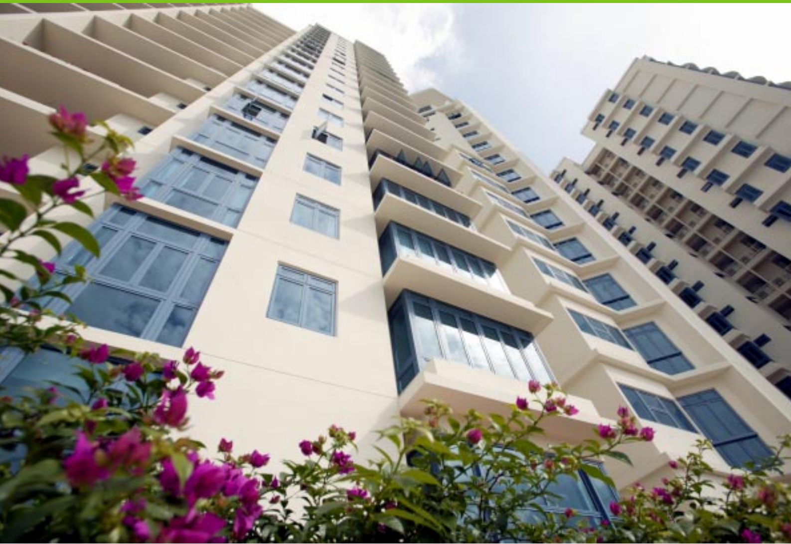
Excellent surface and alignment achieved through precast construction.
