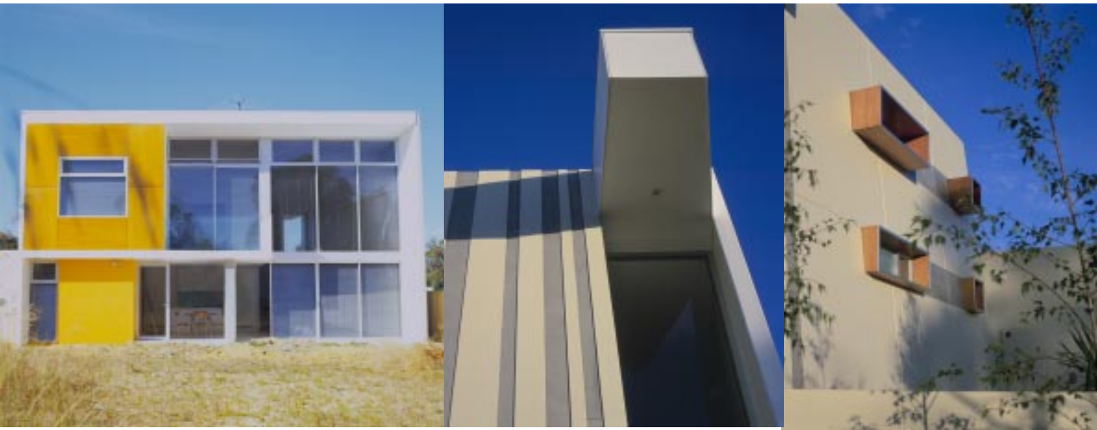
(From left) Rear north-facing façade has extensive glazing with protective overhangs; Vertical recessed bands were used as a graphic device and cast into the panel at the front entrance; Front façade detail showing timber window brise-soleil.
