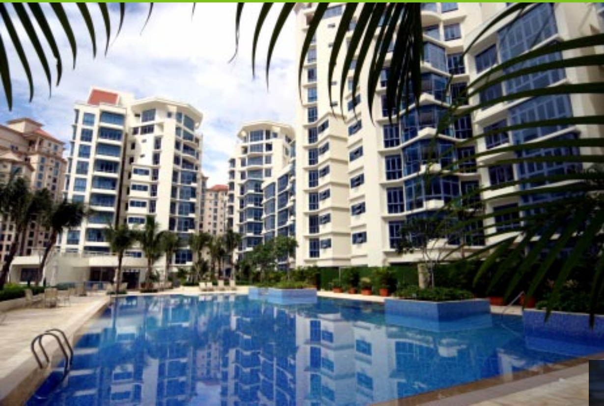
View from the pool. Interplay of circular and triangular precast balconies with octagonal roofs provides exciting variations to the façade.
