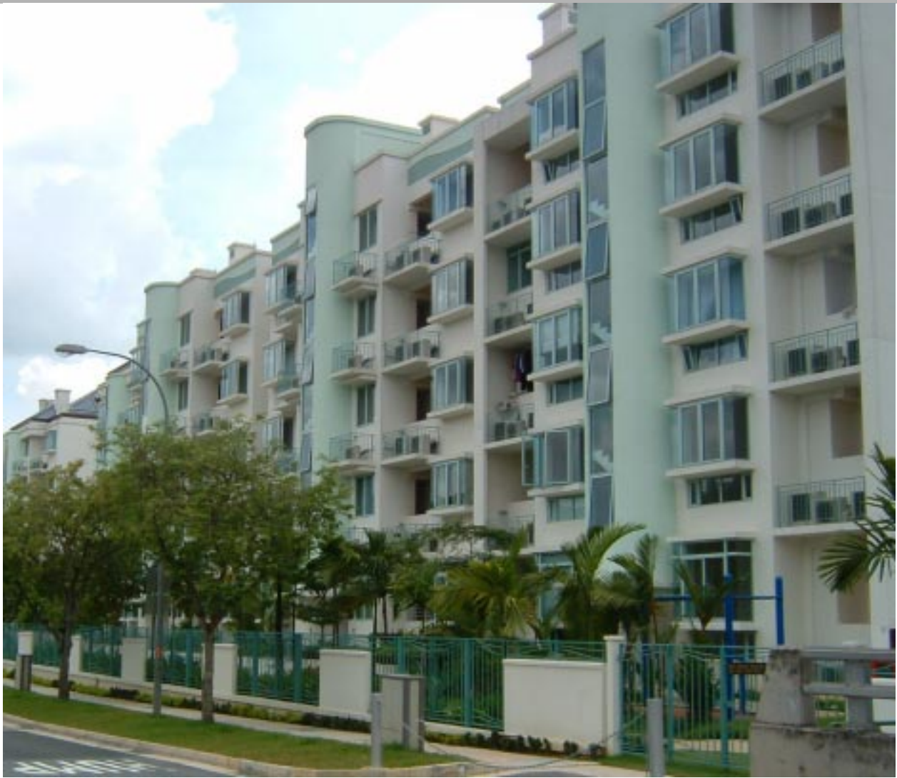
Curved precast staircase wall along Sunset Way.
