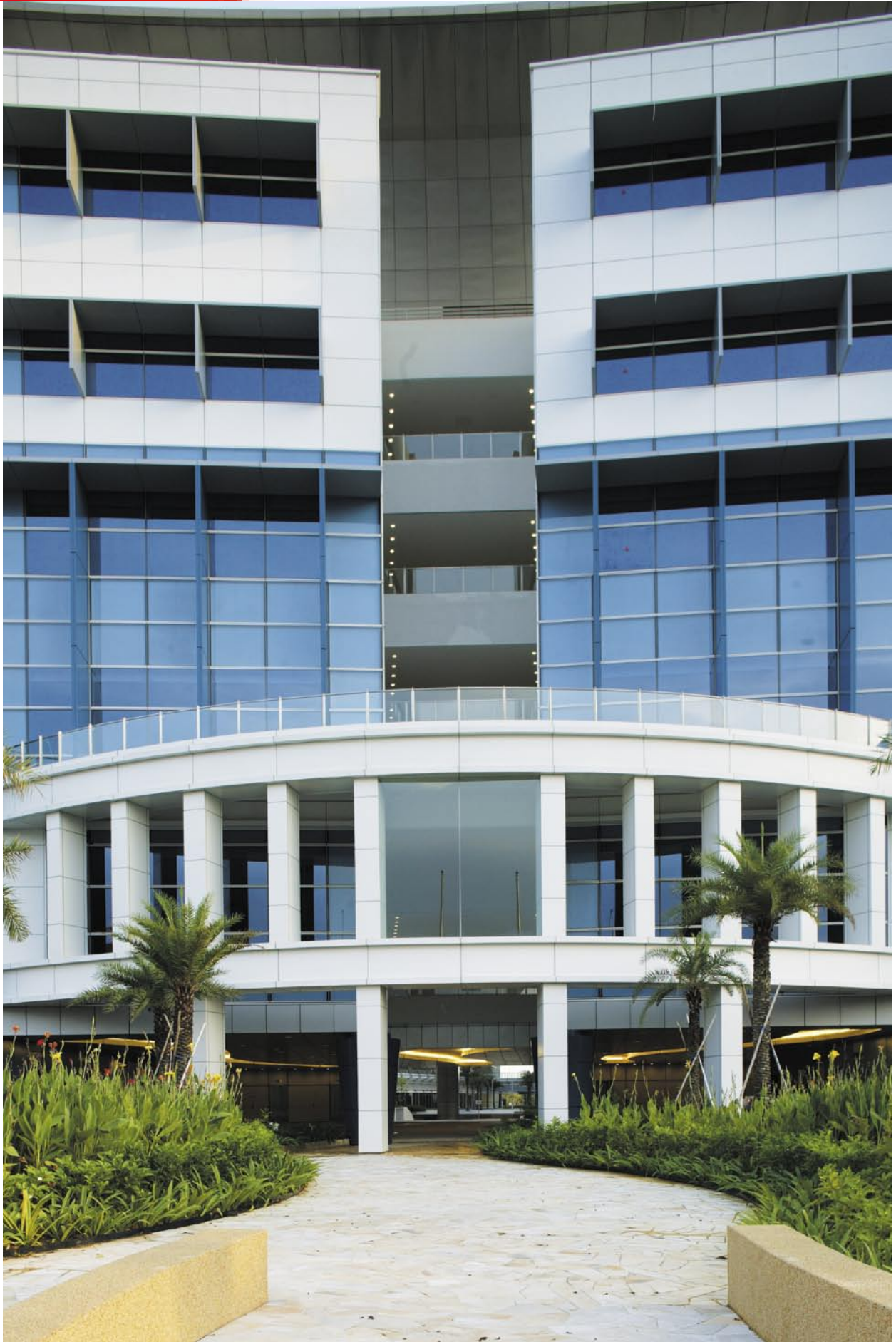
Curtain wall façade at the entrance to Technology Block
