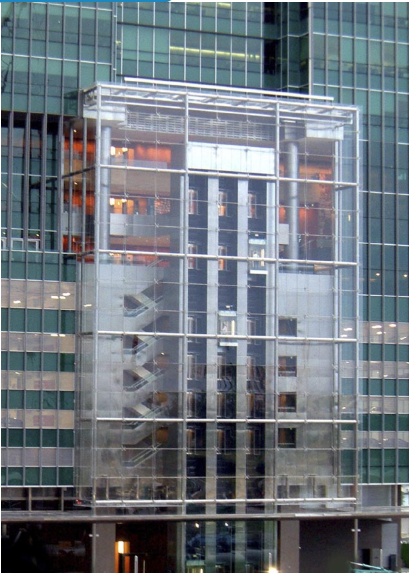
Glass box enclosing carpark lift lobby
