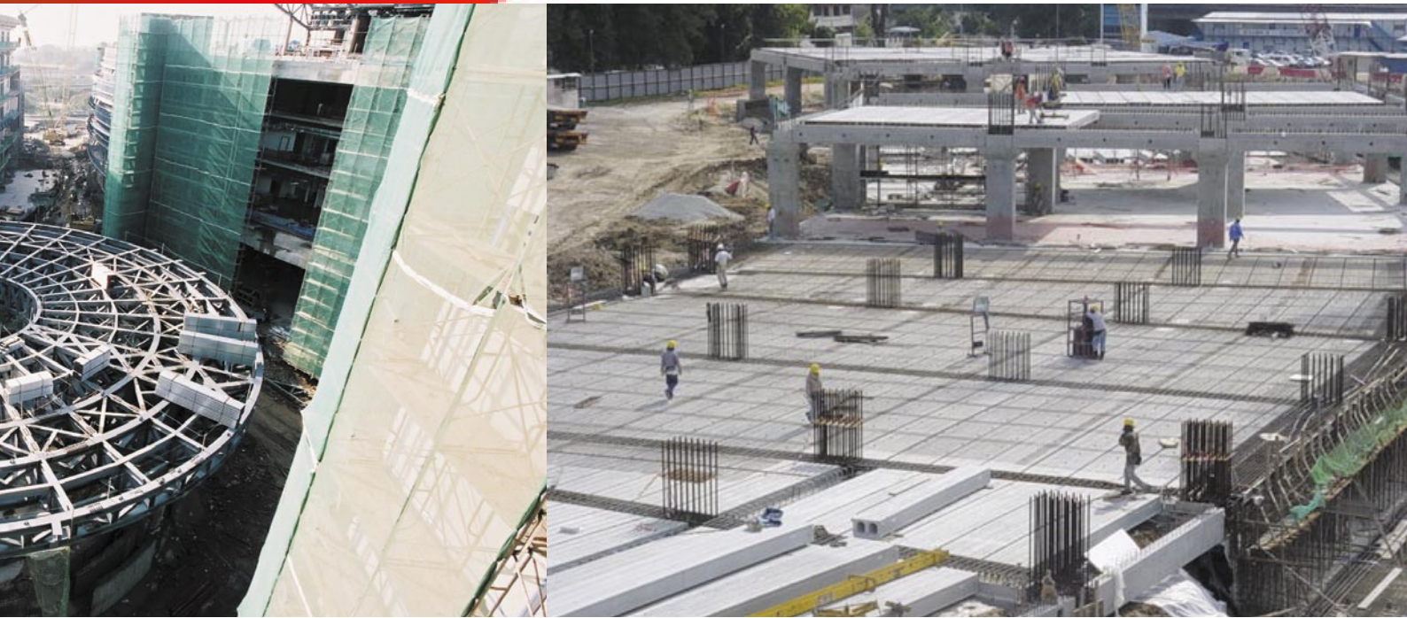
Construction of precast structures
