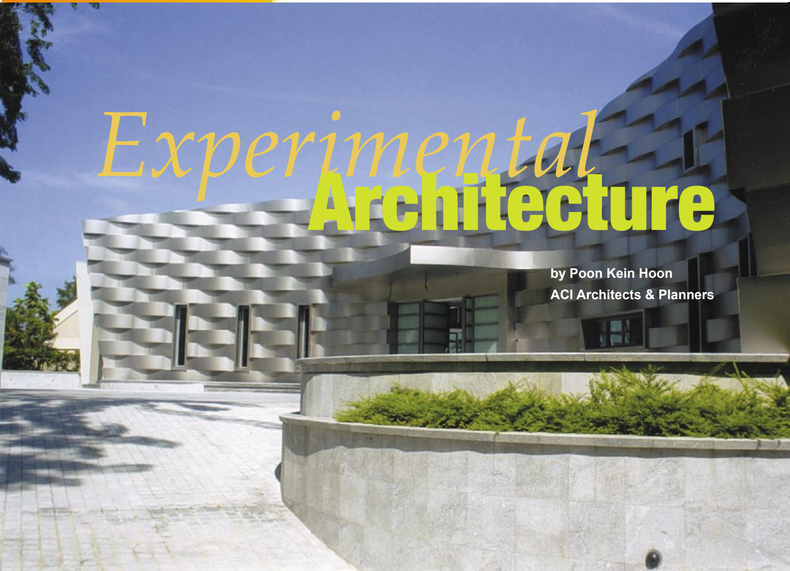
The titanium woven ribbon facade at the front porch with ramp leading to the semi basement
