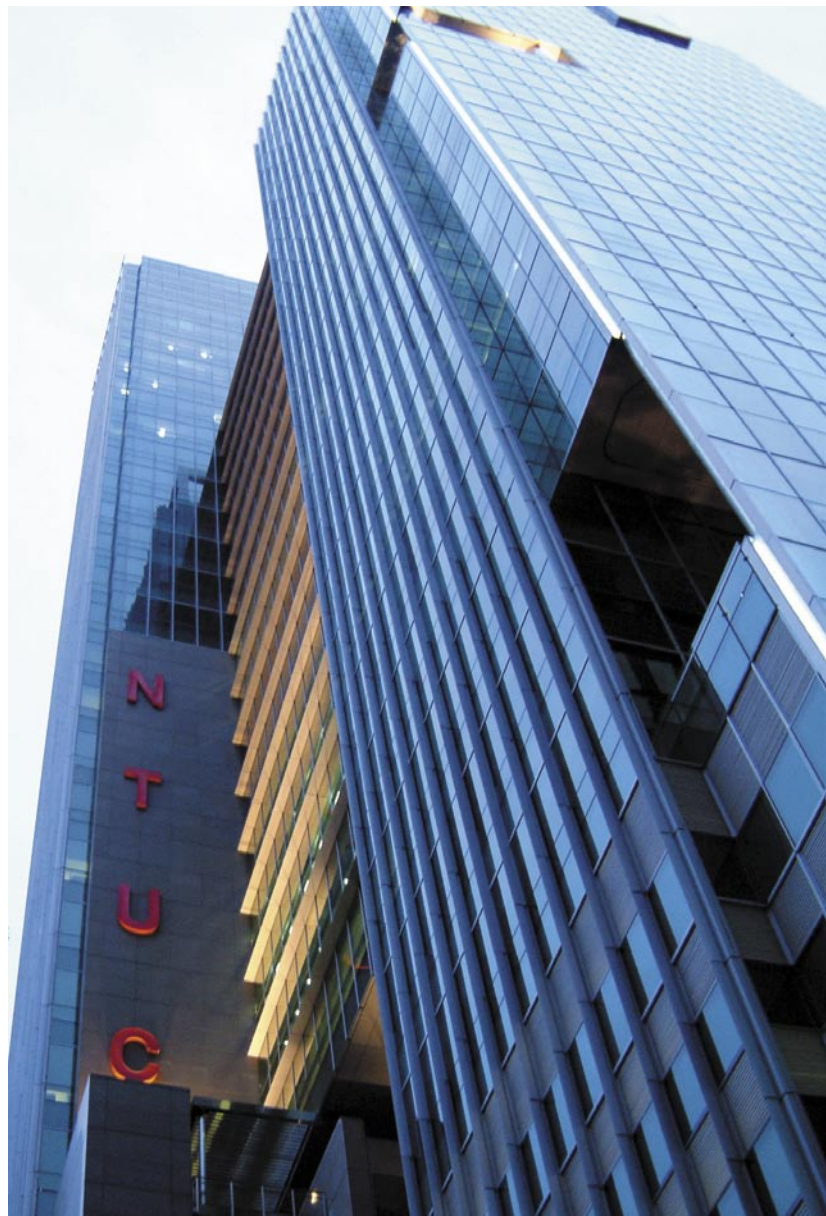
The façade comprises a combination of glass, aluminium and granite panels
