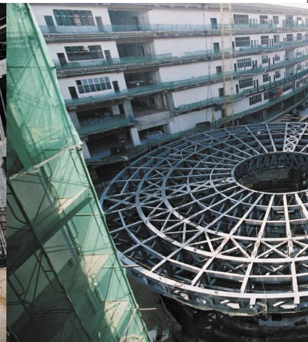
Construction of Forum steel structure
