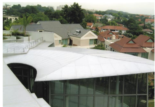
Extensive use of prefabricated metal roof
