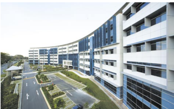
Facade articulation of curtain wall, aluminium cladding and sunshading fins
