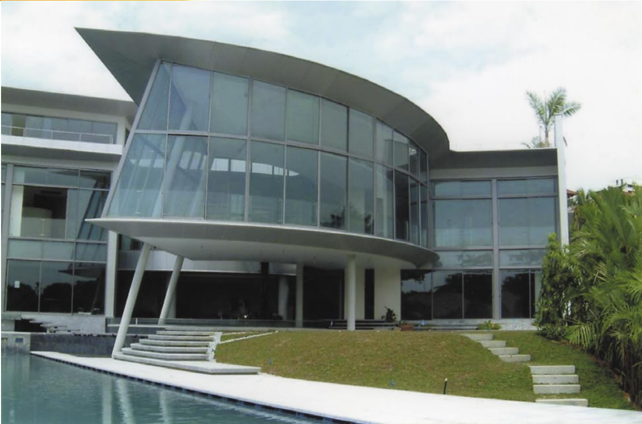
The elevated and ark-like living room
