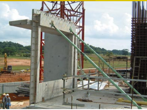
Erection of facade wall with integrated air-con ledge
