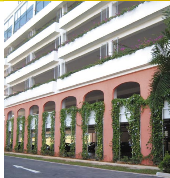
Two-storey high precast arches at multi-storey carpark facade
