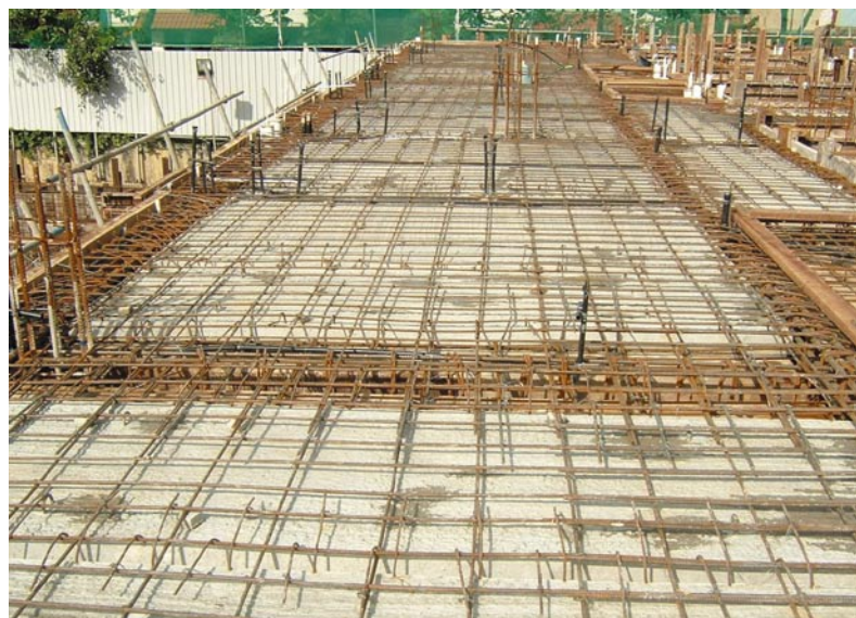
Precast planks at 2nd storey
