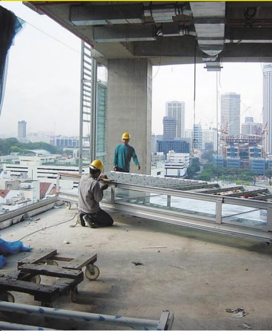
Preparing for the installation of the unitised curtain wall
