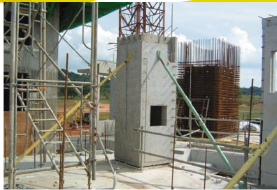
Installation of precast refuse chute
