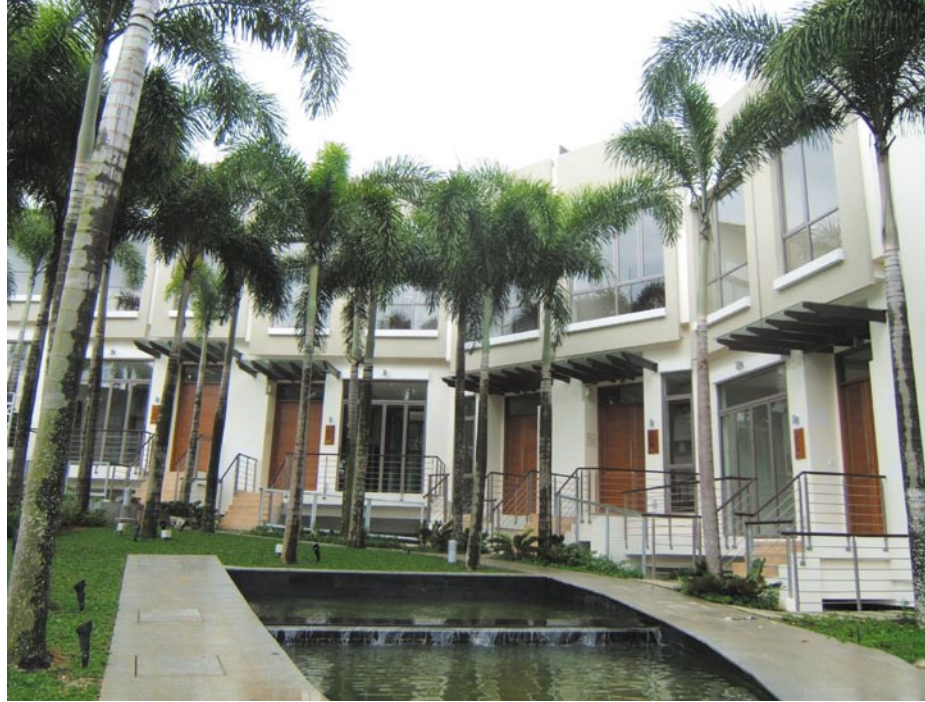
Front elevation of precast panels, large windows and timber trellis
