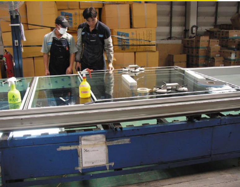
Fabrication of unitised curtain wall in overseas factory
