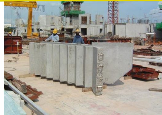
Prefabricated staircase structure
