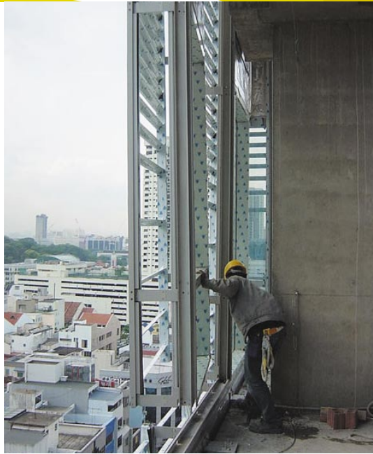
Installation of the unitised curtain wall
