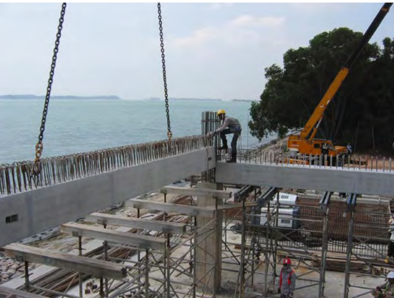
Drop-Off Porch showing the Spider Clamp Point Supports
