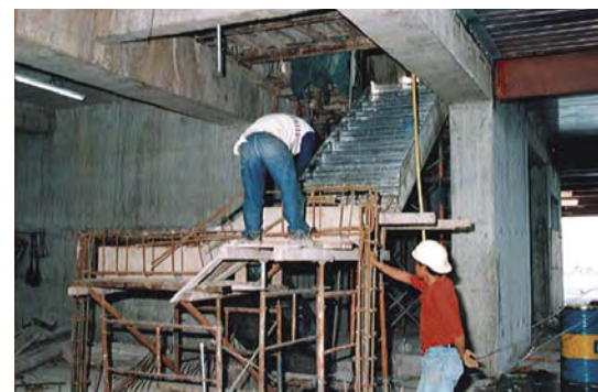
Stairmaster system using standardised pre-assembled steel staircase system
