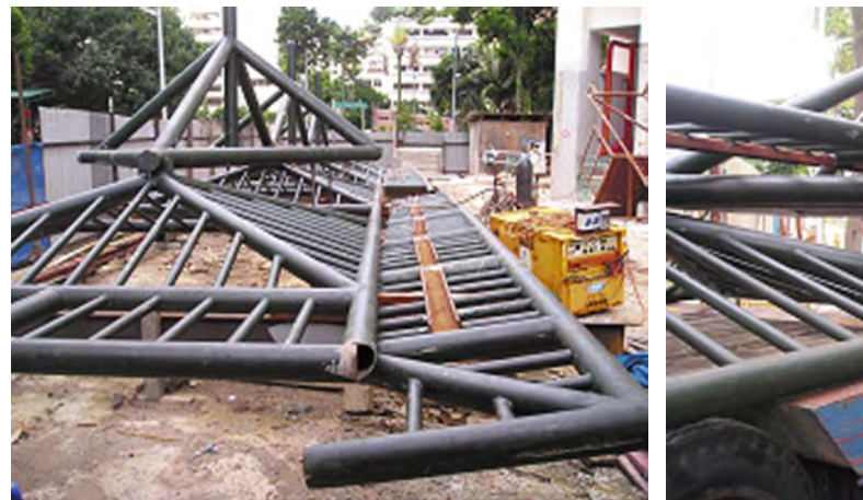
Steel feature at roof level
