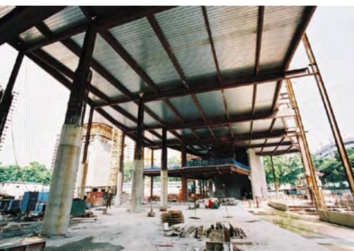
Composite steel beams with bondek slab were used for erection purpose
