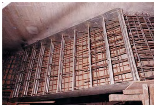
Stairmaster system using standardised pre-assembled steel staircase system
