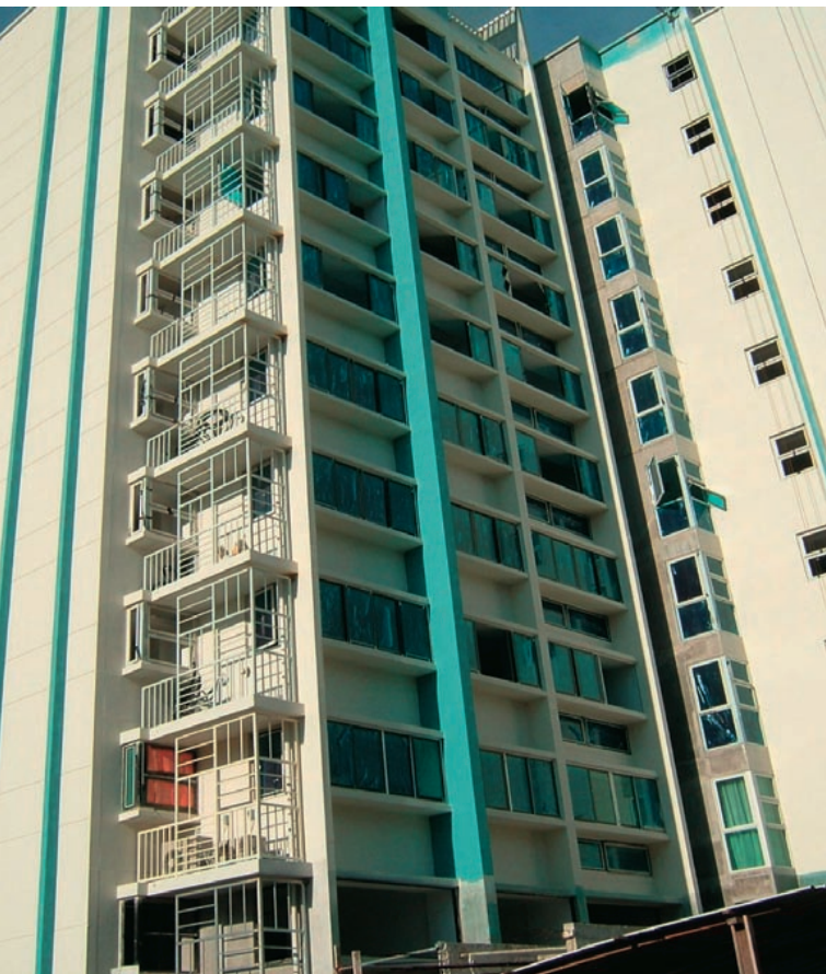
Close-up of precast facade
