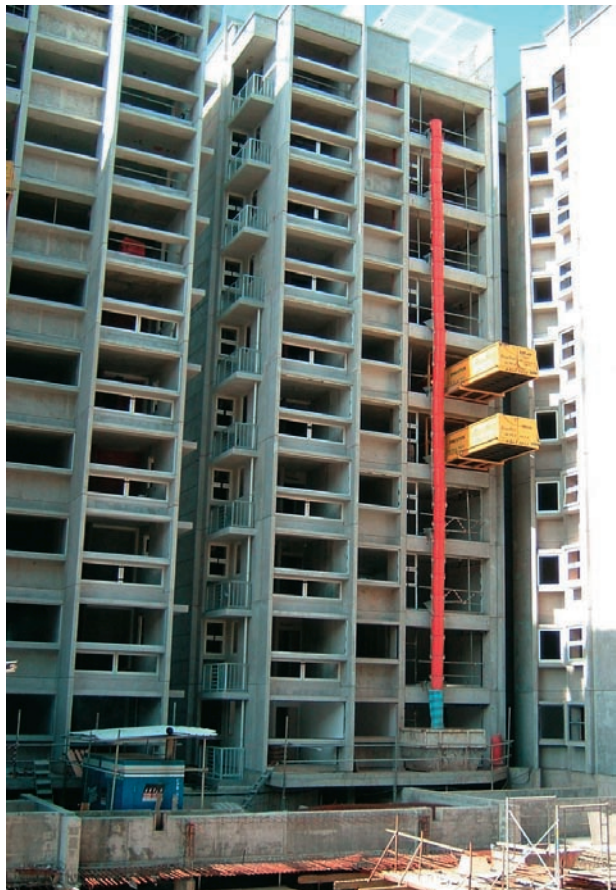
Scaffoldless construction site
