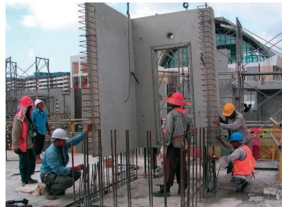
Installation of precast household shelter
