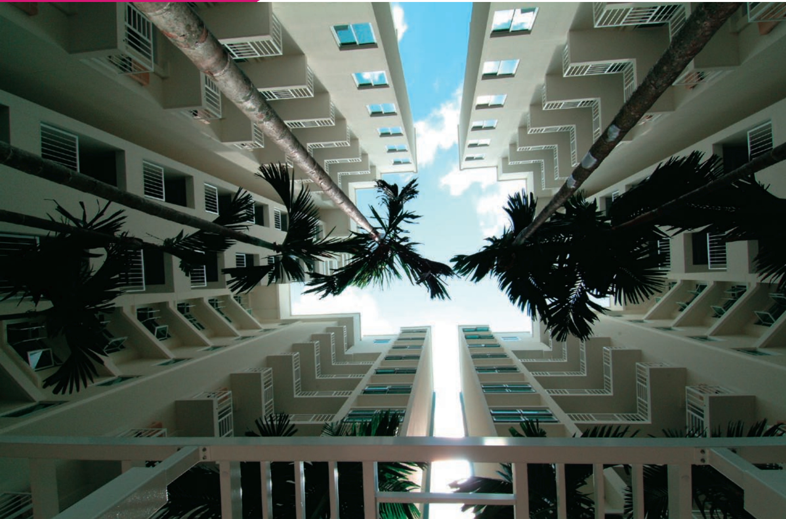
Elegant view of precast components
