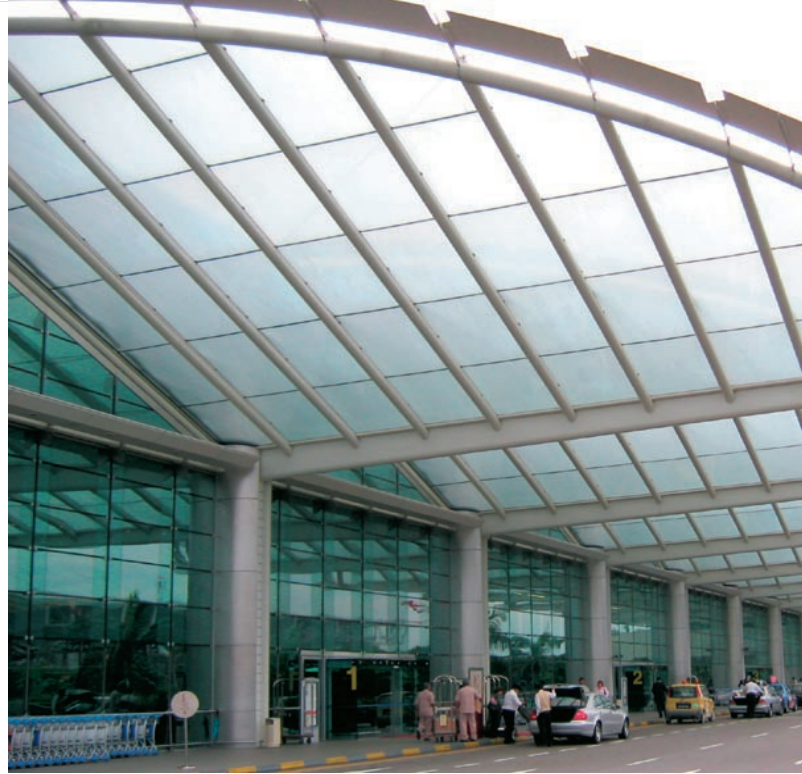
The prominent entrance canopy and curtain wall facade
