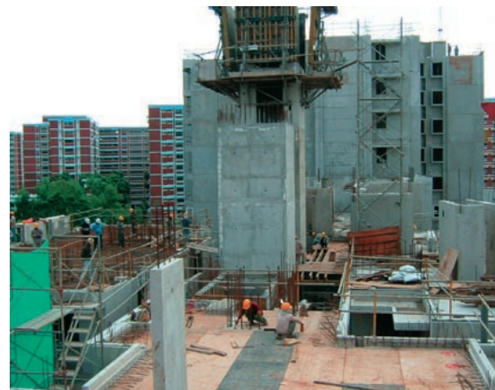
Installation of vertical precast elements
