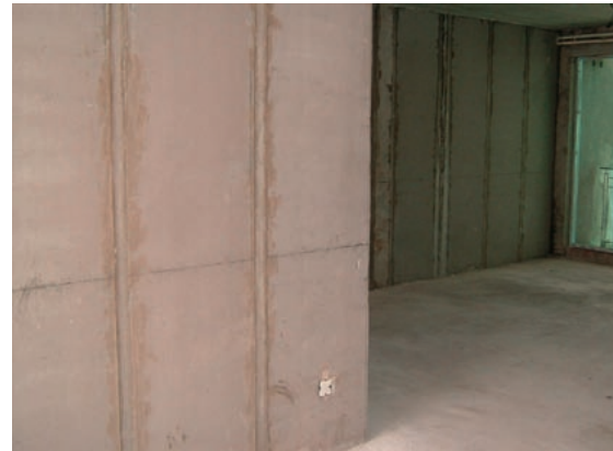
Using lightweight precast concrete panel as interior wall
