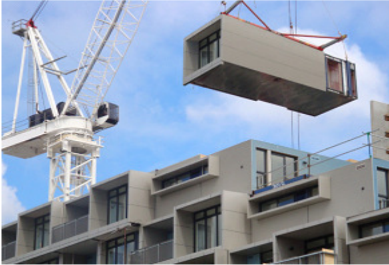
PPVC installation on site – Picture courtesy of UB Australia
