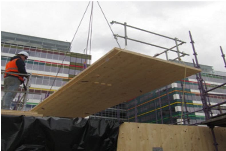
CLT installation on site – Picture courtesy of Lend Lease
