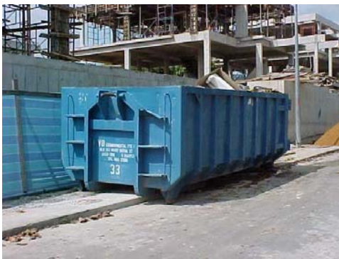
Skip on sidewalk - obstruct pedestrians
