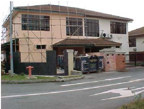
Skip placed within work site - A good practice
