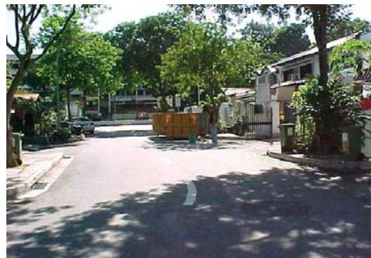
Incorrect retroreflective sheeting - increase risk of accident
