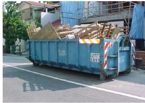
Skip as temporary storage space - Road users at risk
