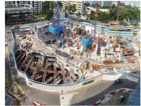
Actual installation of tower cranes on site
