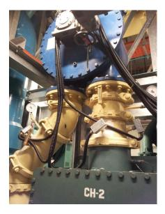
All the new chillers in Keppel Bay Tower will be equipped with auto tube cleaning system which is effective in maintaining the cleanliness and the efficiency of the chiller condenser heat exchanger.
