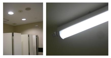
Motion sensors are installed in toilets and staircases to reduce energy use as well as lengthen the operational life of the light-fittings and bulbs.
