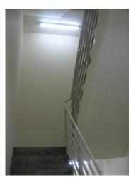
LED lightings are installed at the carpark and all staircases within Keppel Bay Tower. LED lights not only consume less electricity, it also generates less heat, lower carbon emissions, extend maintenance cycles and at the same time, enhance the lighting of the carpark and staircases.
