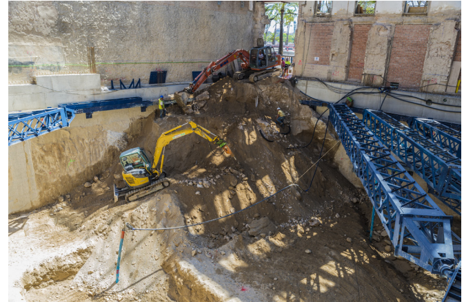
Deep excavation & ERSS. Activities such as deep excavation and ERSS involves more risk due many considerations including safety, accessibility of equipment to excavated levels, complexity of the methodology, among many others.
