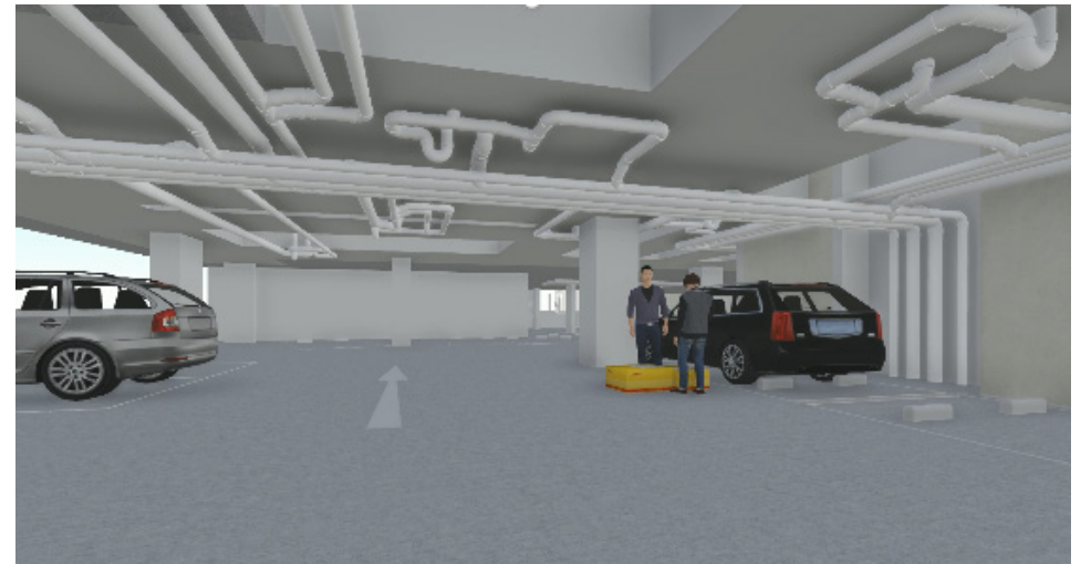
Headroom requirements. Check for headroom requirement and visual arrangement of services in public and exposed areas such as basement car parks.
