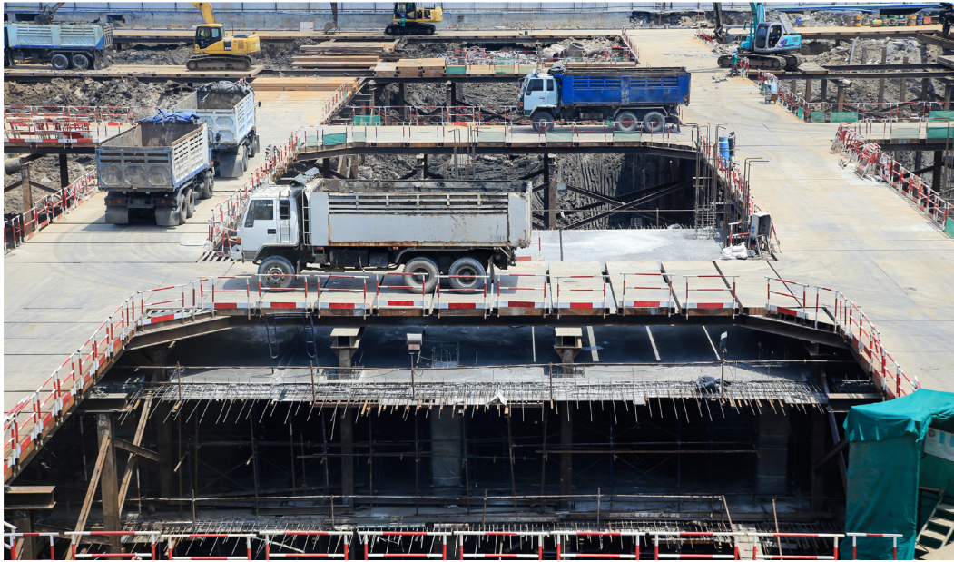
Deep excavation & ERSS. Activities such as deep excavation and ERSS involves more risk due many considerations including safety, accessibility of equipment to excavated levels, complexity of the methodology, among many others.
