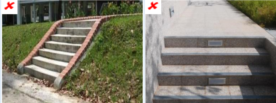
Figure E—XI: Photos from site inspections that depict staircase which are not provided with handrail
