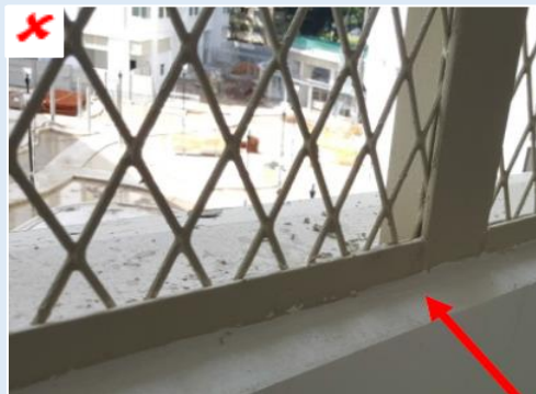
Figure H—XII: An example of a toehold at a protrusion > 50mm width
