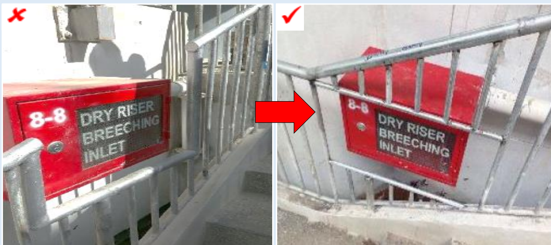
Figure E—XVI: Non-continuous handrail due to MEP fixture
