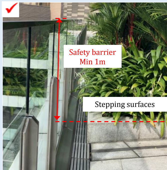
Figure H—XIV: Minimum safety barrier height of 1m from stepping surfaces
