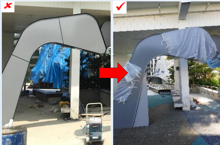
Figure C—VIII: Slanted structure at gym area is straightened
