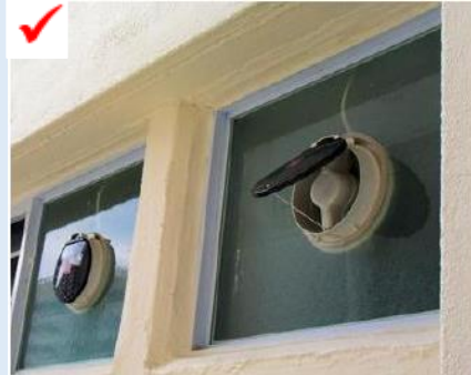
Figure G—I: Window or Wall mounted fan
