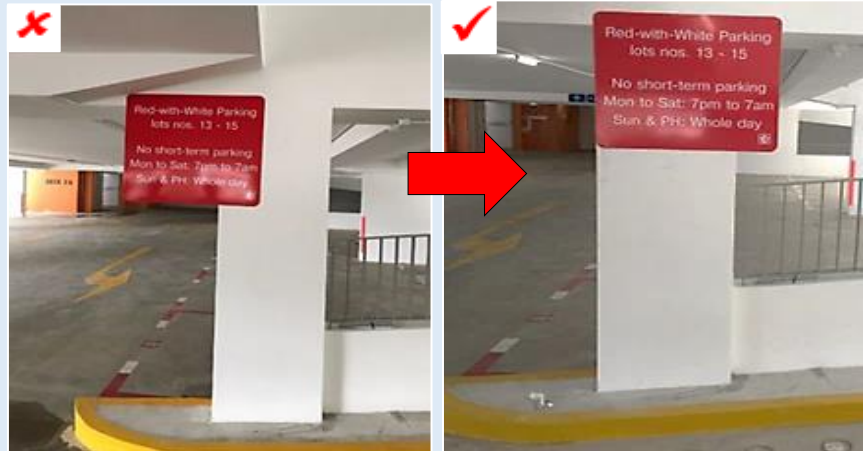
Figure C—IV: Change of location of signage to meet headroom requirements
