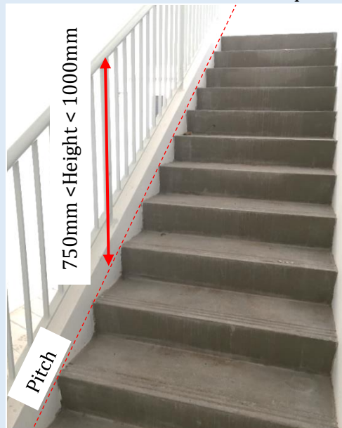
Figure E—XII: An example on the measurement of height of handrail from the pitch line
