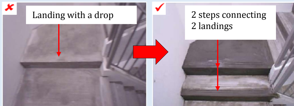
Figure E—IX: An example of landing with a step being rectified
