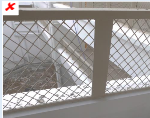
Figure H—XI: Climbable toehold of a perforated barrier
