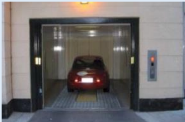
Figure K—I: Car lift intended to convey vehicles together with driver/passengers
