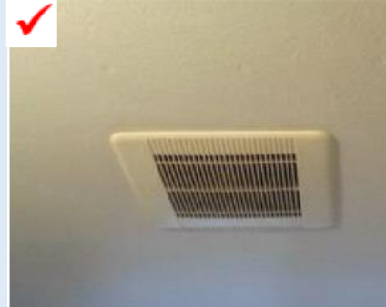
Figure G—II: Ducted fresh air supply outlet
