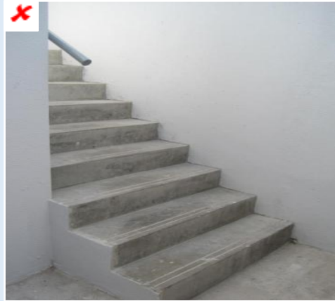
Figure E—XV: Non-continuous handrail
