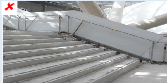
Figure E—V: Incomplete finishing work
