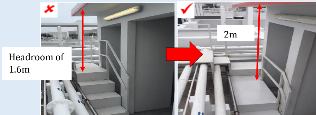
Figure C—V: Steel staircase was rectified to increase headroom space
