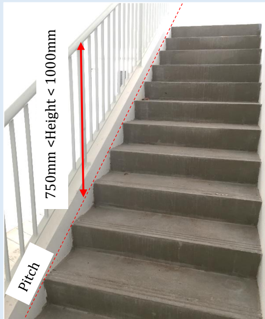
Figure I: An example on measuring height of handrail from pitch line
