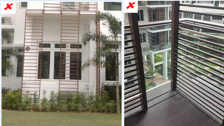
Figure H—III: The horizontal members create a ladder effect tempting children to climb and expose them to risk of falling from height
