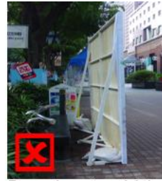
Exposed counterweight/ sandbags & brackets
