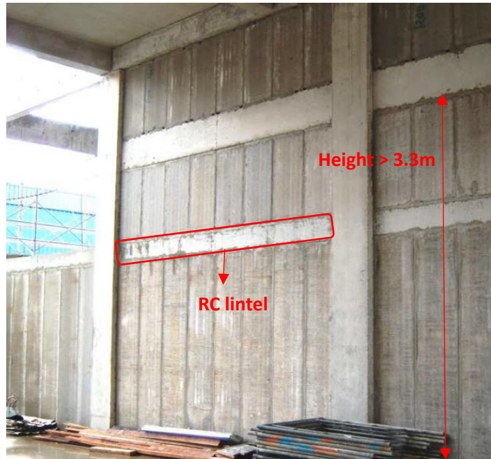
Figure 3: Erected precast hollow concrete wall with RC lintels
