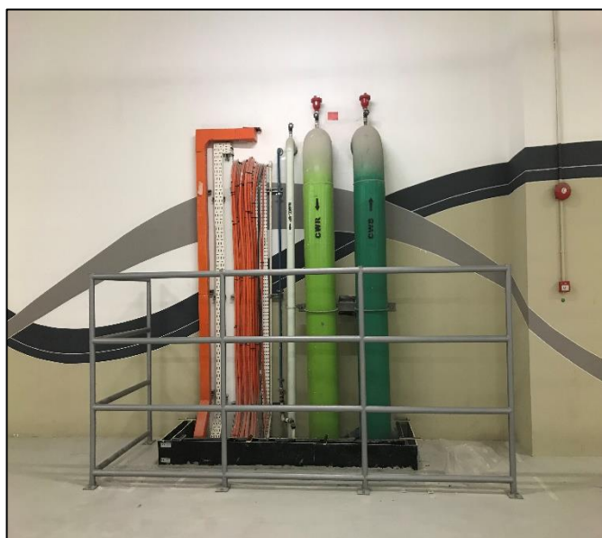
Example of dedicated shafts for pipes/cables
