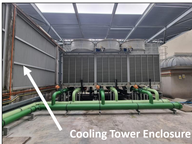
Example of the Cooling Tower Enclosure
