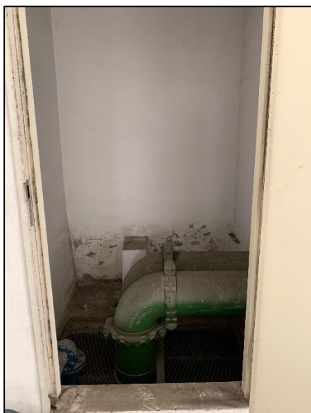
Example of dedicated shafts for pipes/cables
