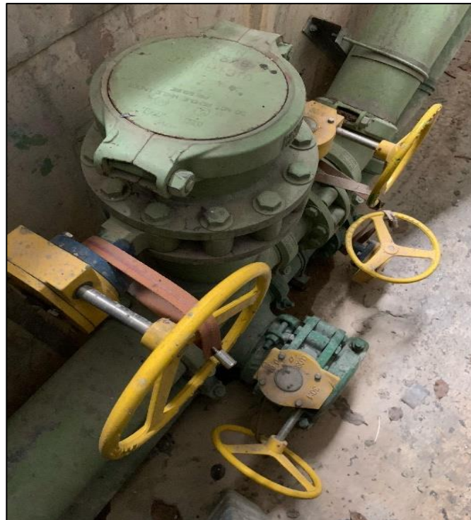
Example of pipe tee joint for chilled water pipes
