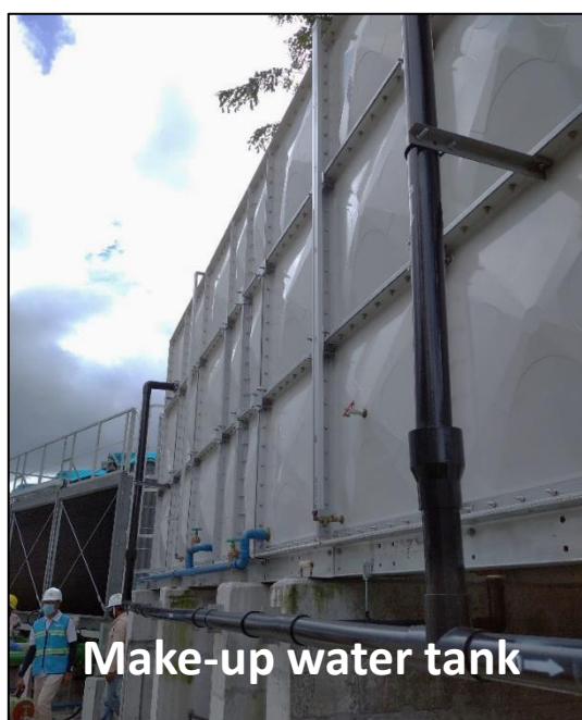
Example of RTS Cooling Tower and Make-up Water Tank
