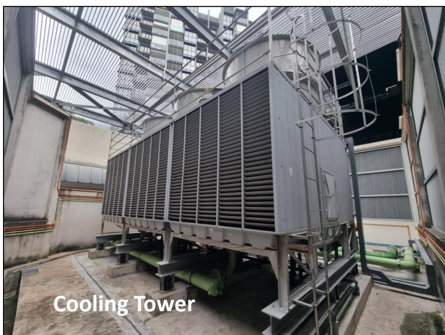
Example of RTS Cooling Tower and Make-up Water Tank
